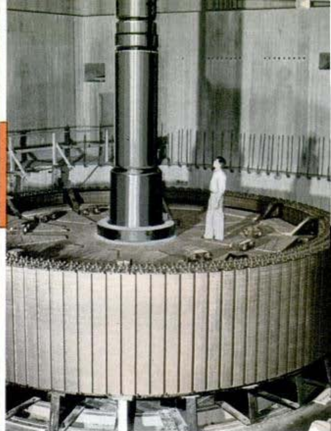
Rotor for one of the Grand Coulee generators weighs 587 tons and is 31 feet in diameter. Turning at 120 revolutions per minute, the speed of its outer rim is 130 miles an hour
